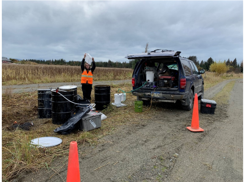
Exhibit 2-2: Monitoring well development; visually checking turbidity.
